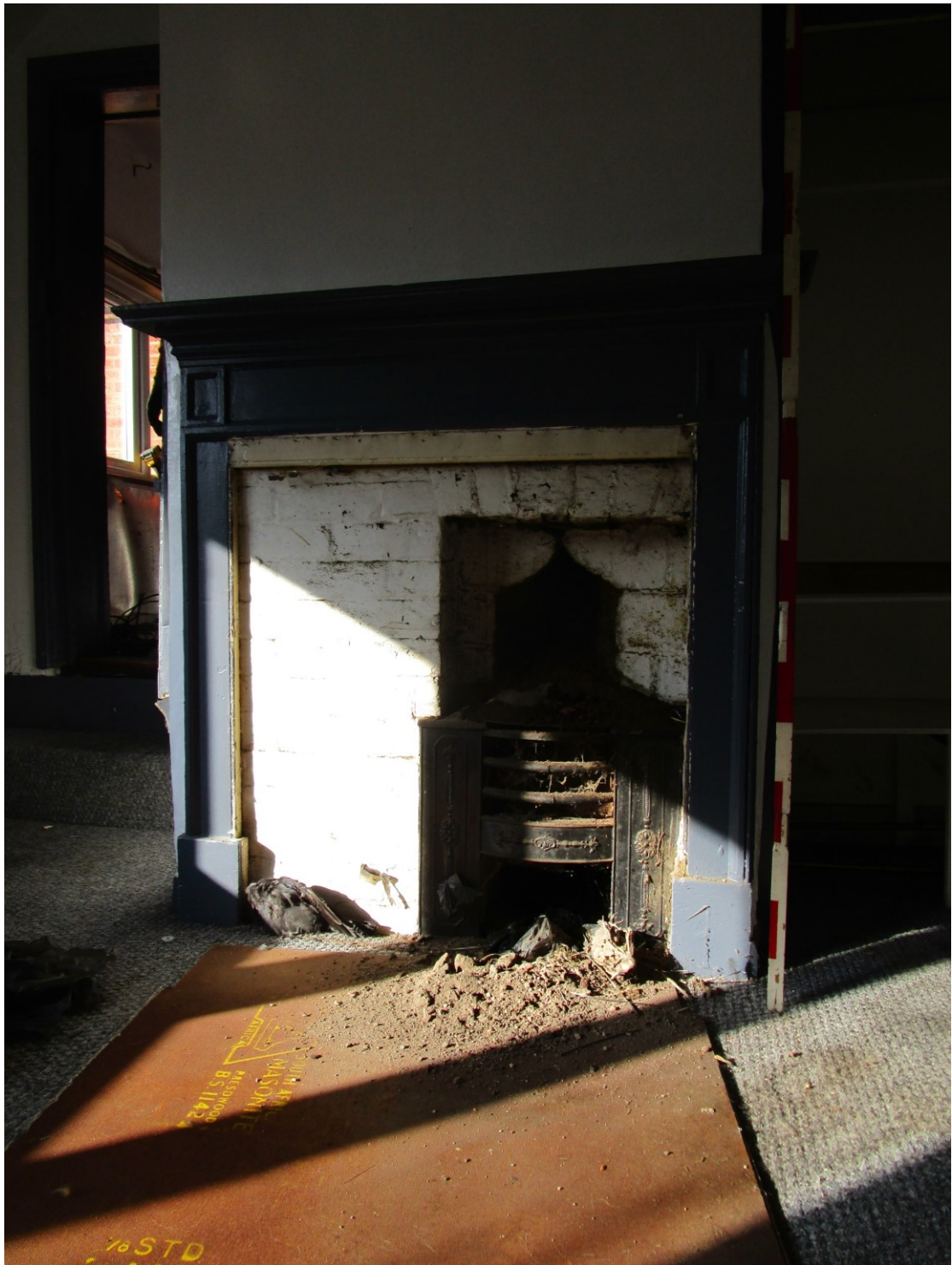
Plate 21; 1st floor fireplace, behind that shown in plate 20, in the rear wing extension. Note the positioning to allow for the flue from the ground floor.
