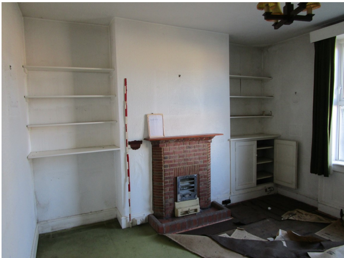
Plate 18; 'Art Deco' fireplace on the ground floor.
