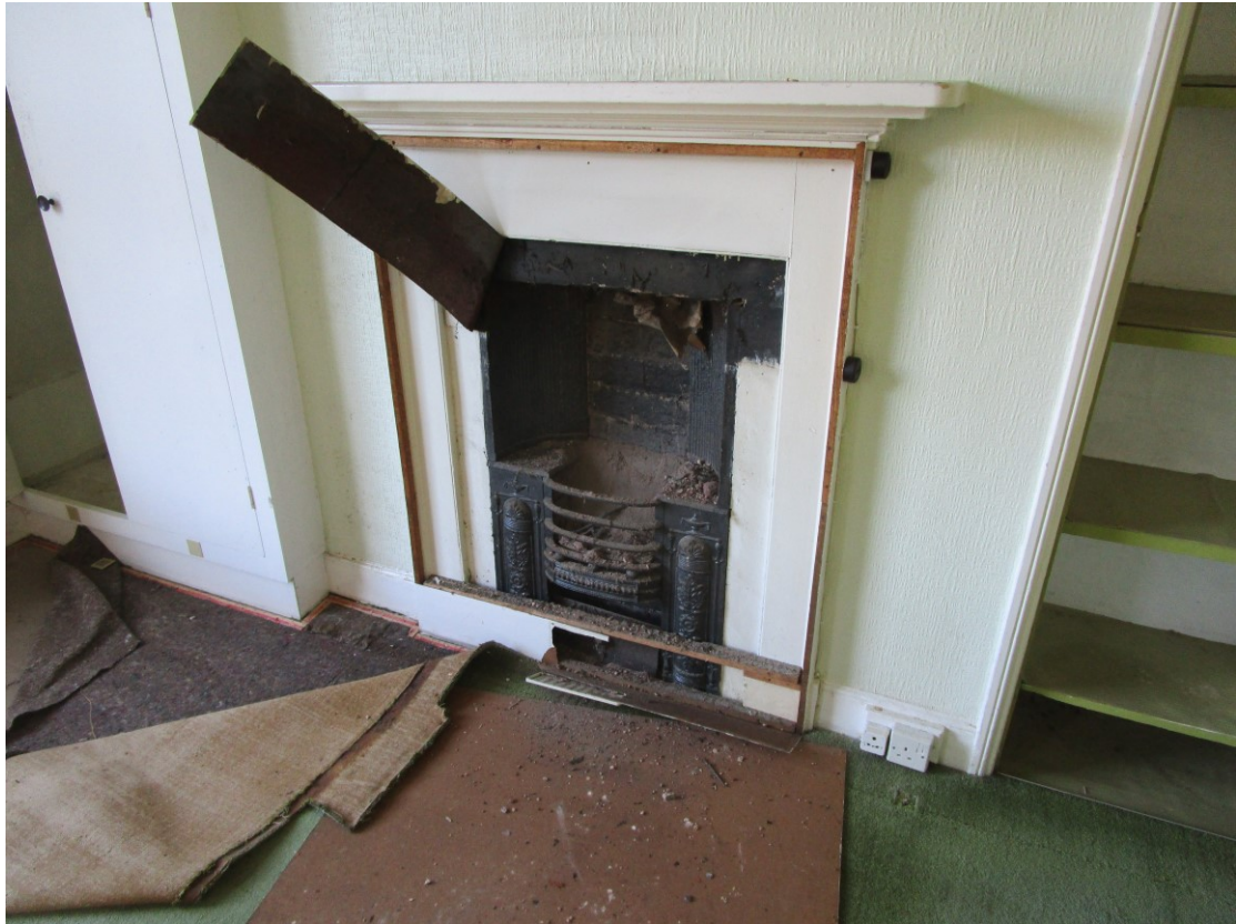
Plate 19; 1st floor fireplace.
