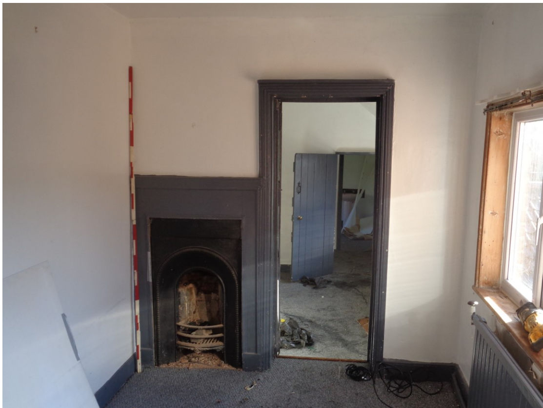
Plate 20; 1st floor fireplace in original rear wing.
