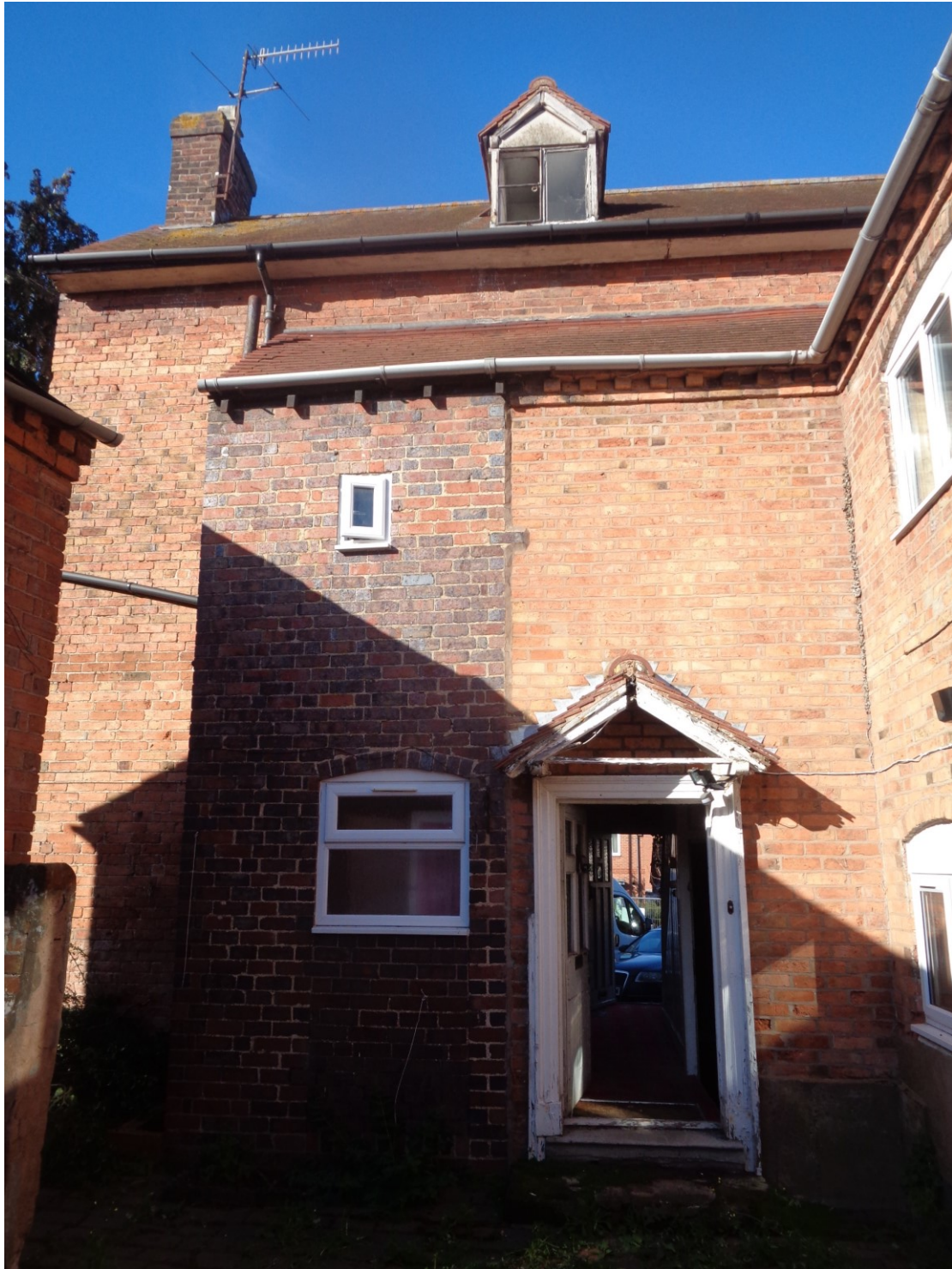
Plate 22; The rear of the main range from the brick-paved yard showing later addition with window inserted into doorway. The dormer window is shared between the stairwell and the adjacent garret chamber.
