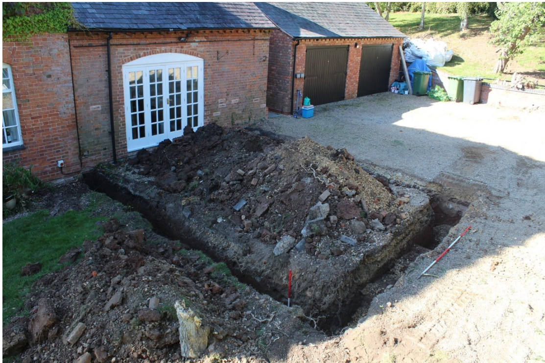
Plate 1; overall view of the foundation trench for the new extension.
