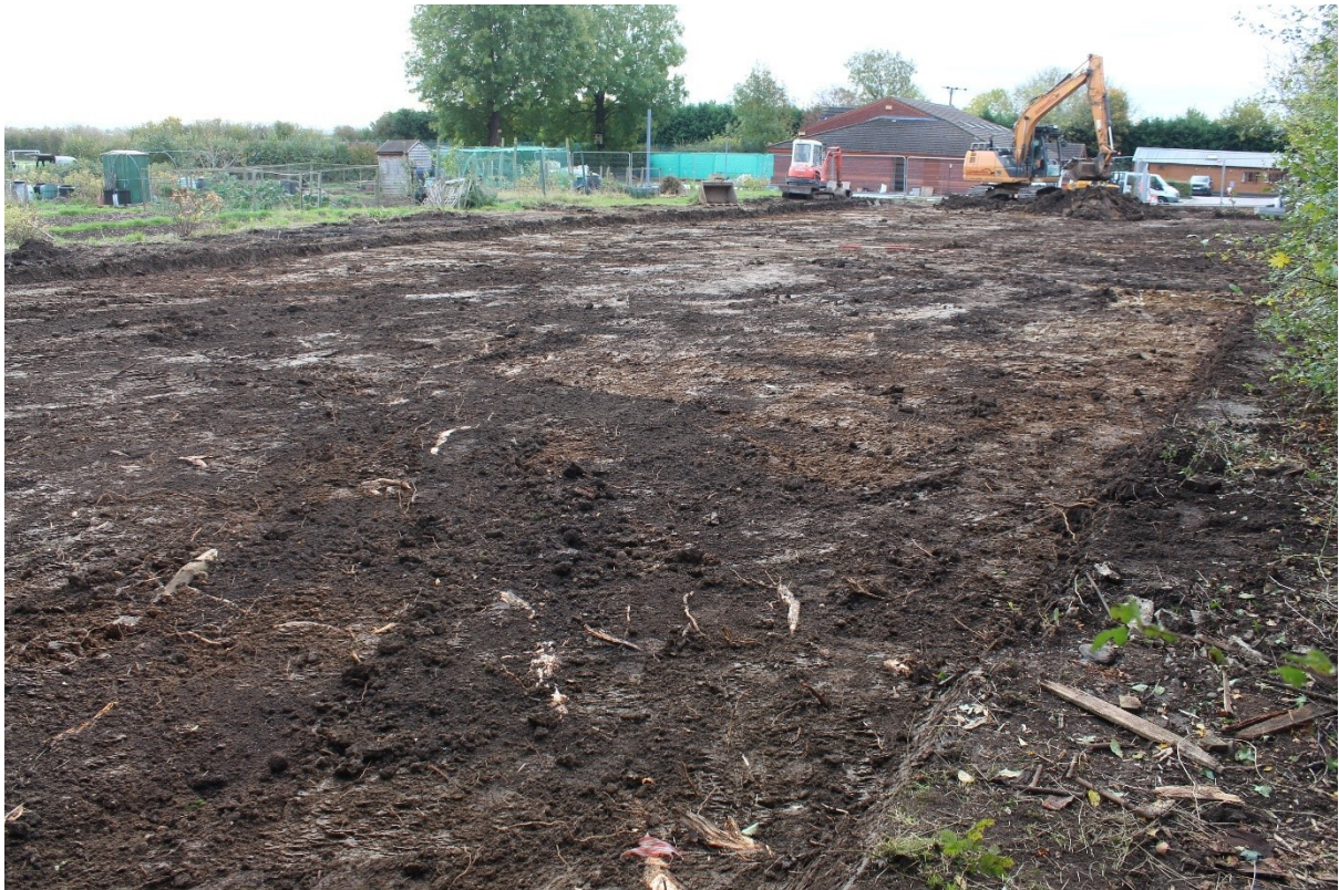
Plate 4; overall view southwest of car park area
