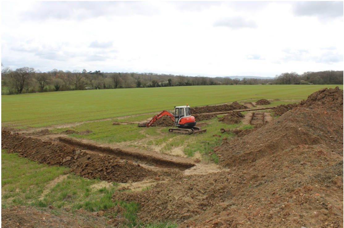
Plate 12: trenches 2-5, overall view southeast
