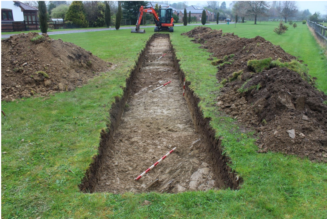
Plate 3: trench 2, view north showing areas of exposed bedrock.
