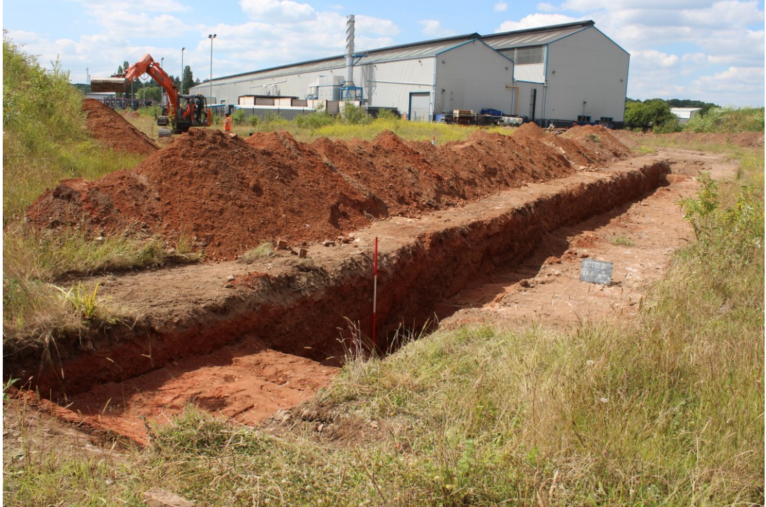
Plate 15: trench 8, view northwest
