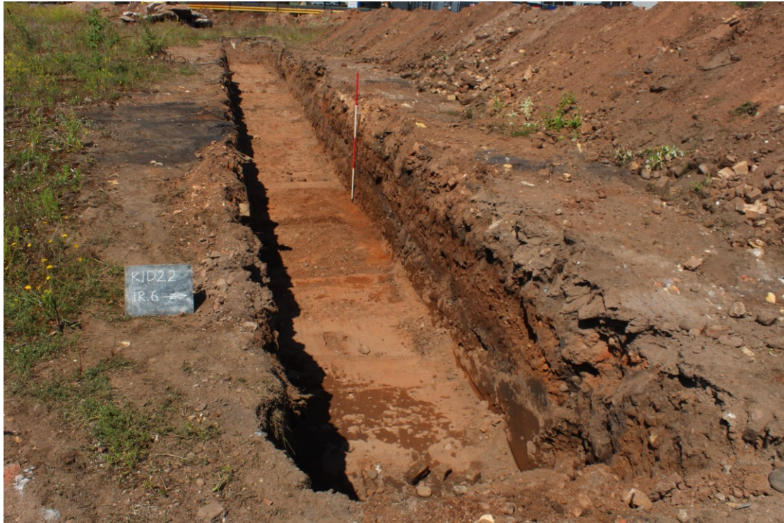
Plate 11: trench 6, view northwest
