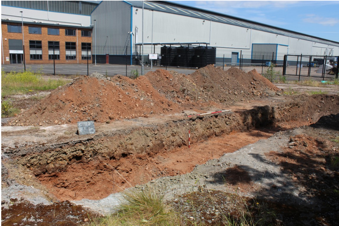
Plate 1: trench 1, view northeast.
