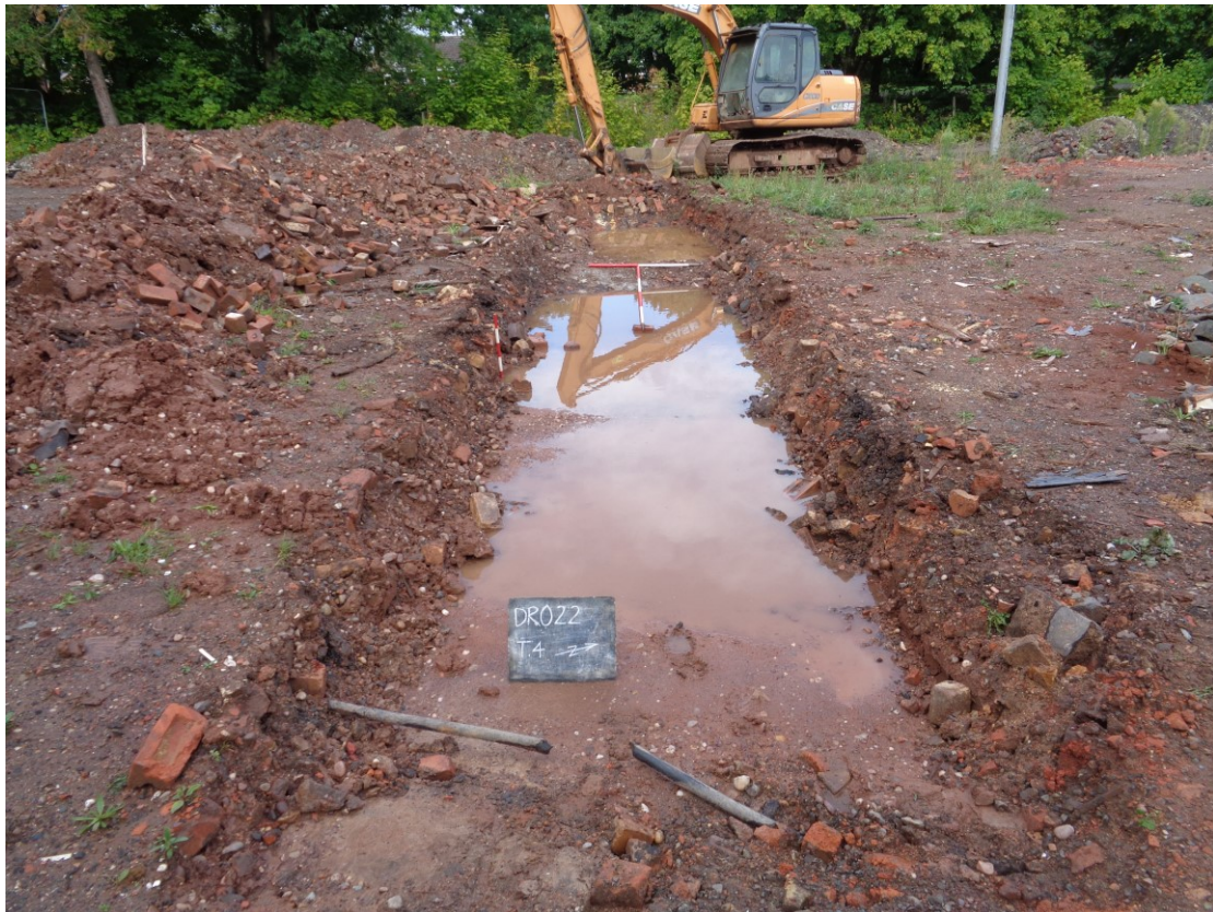
Plate 11: trench 4, view west
