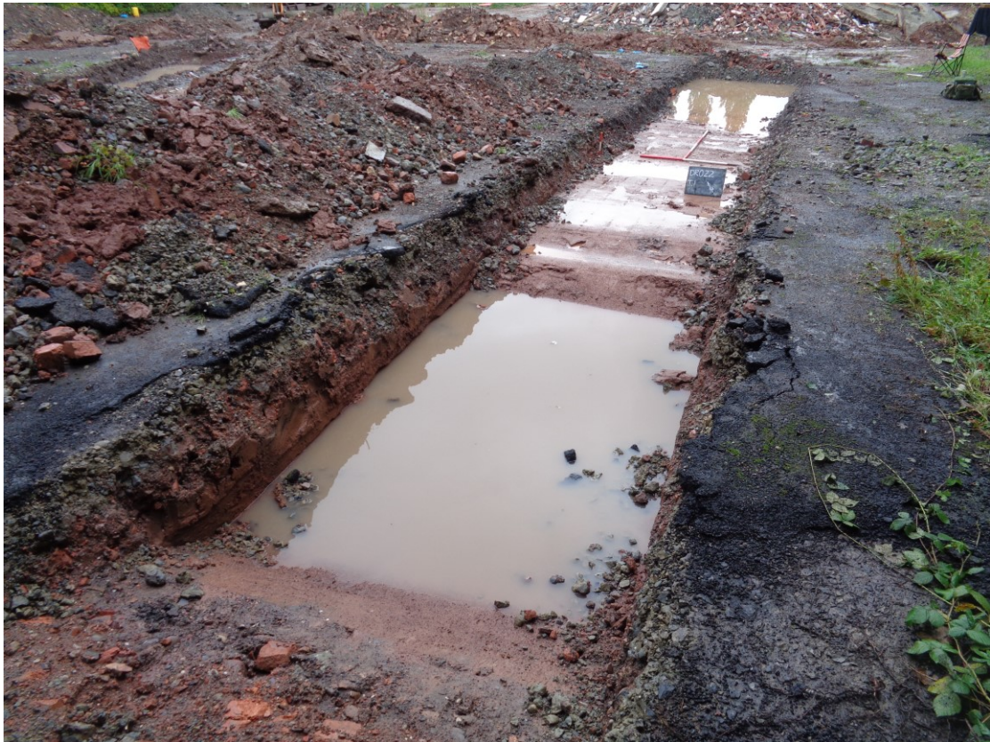
Plate 2: trench 1, view north
