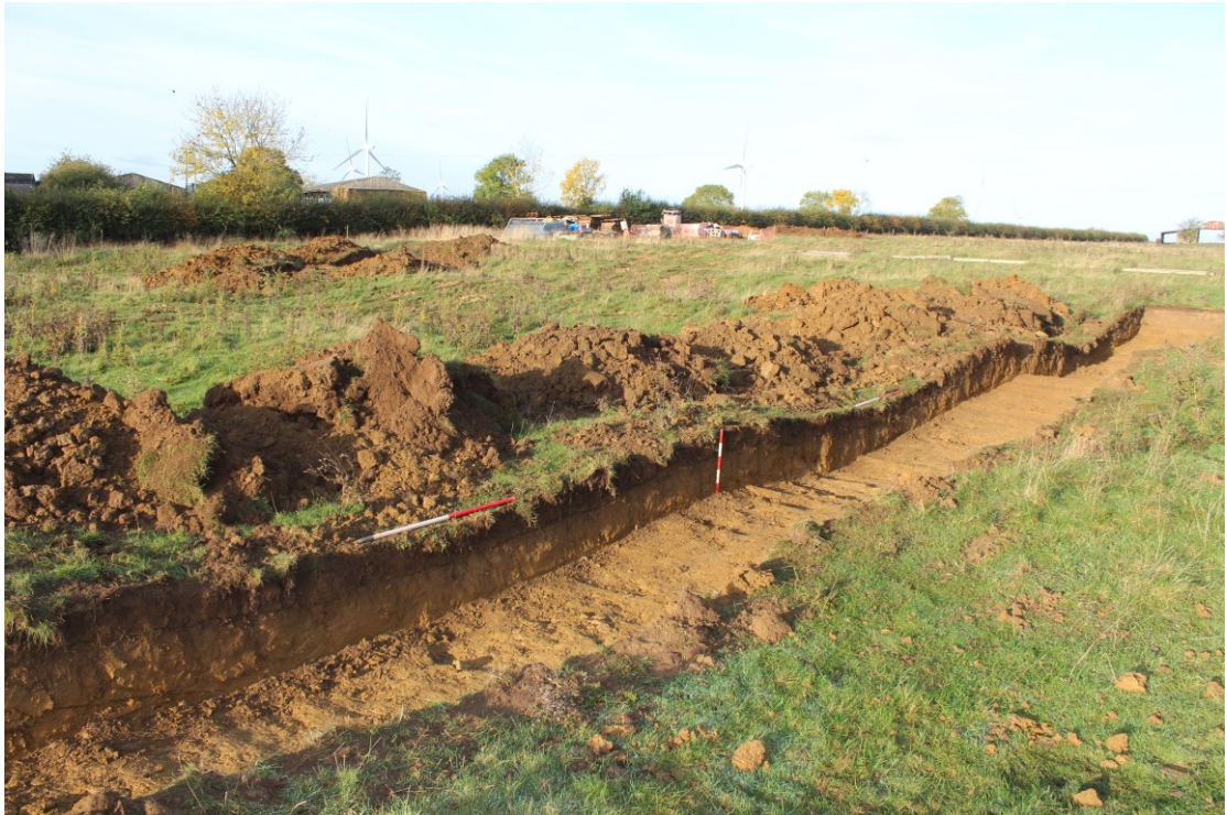
Plate 12: section 4a, view northwest
