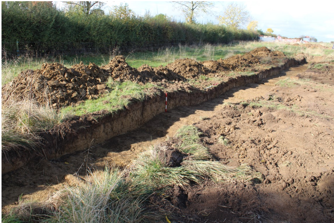
Plate 8: section 2a, view northwest
