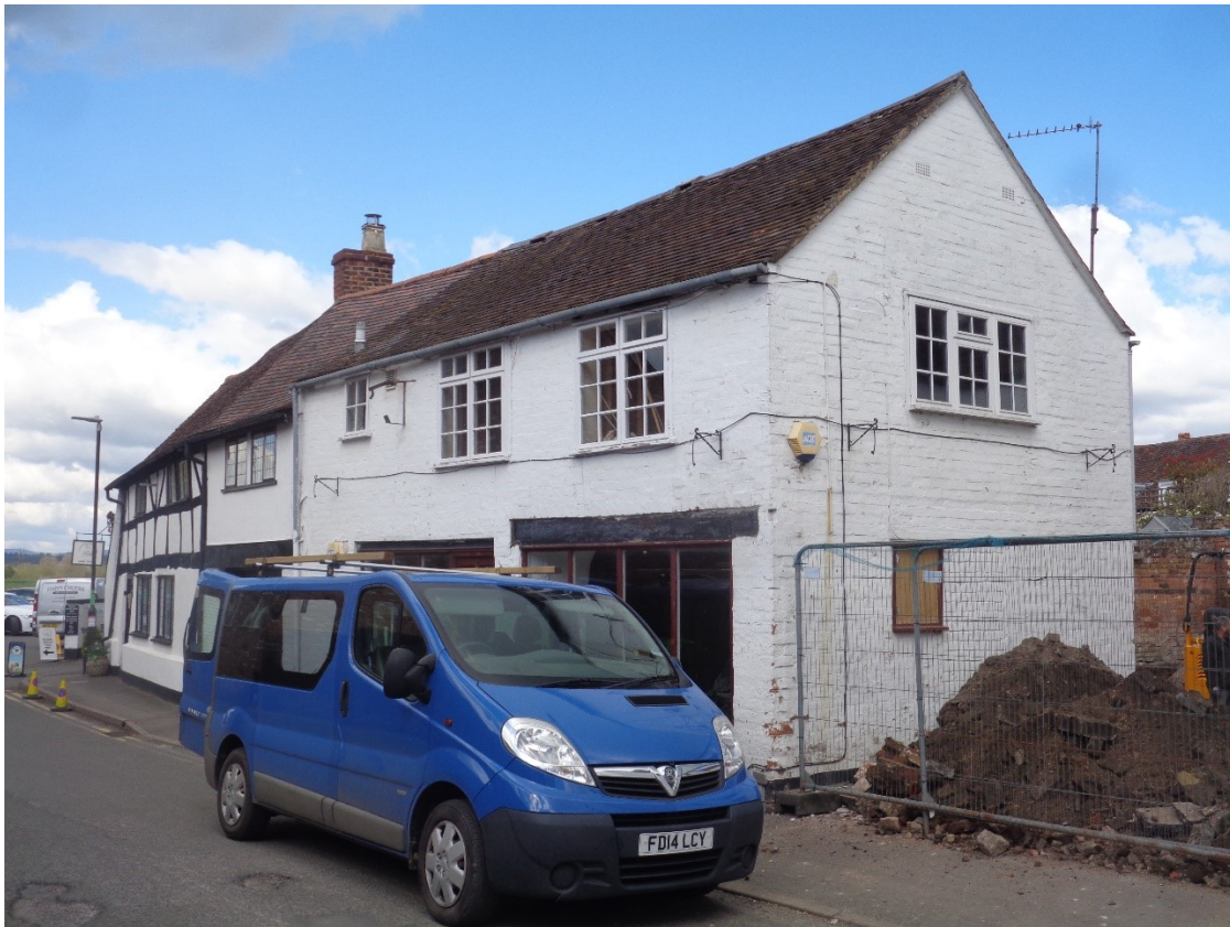
Plate 1; overall view northwest of the property
