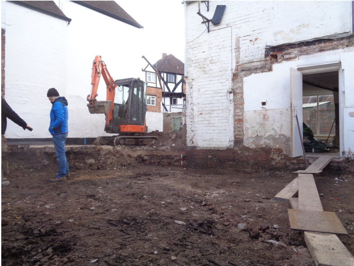
Plate 5; view southeast of the excavation area
