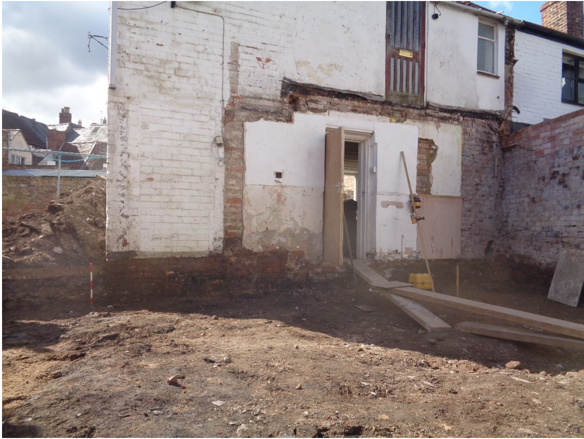
Plate 3; view southwest of the excavation area
