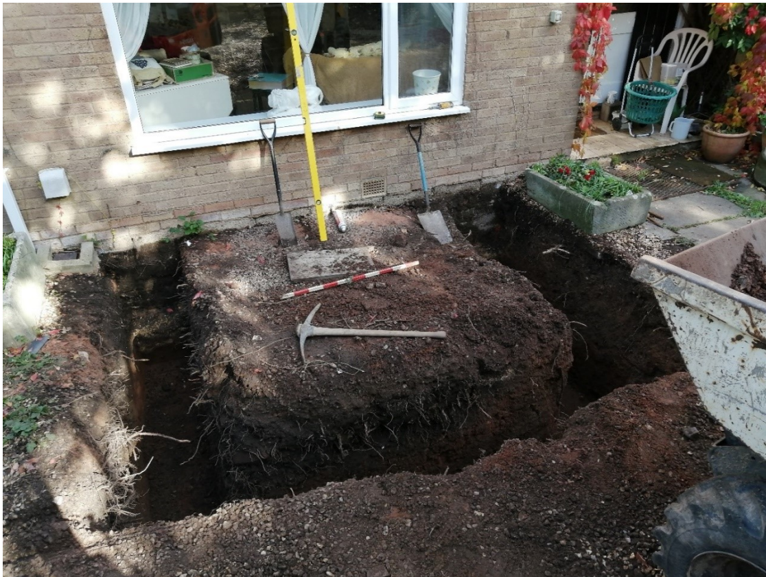
Plate 1: overall view northeast of the foundation trench.
