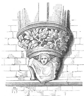
CORBEL OF ONE OF THE ROOF ARCHES.
