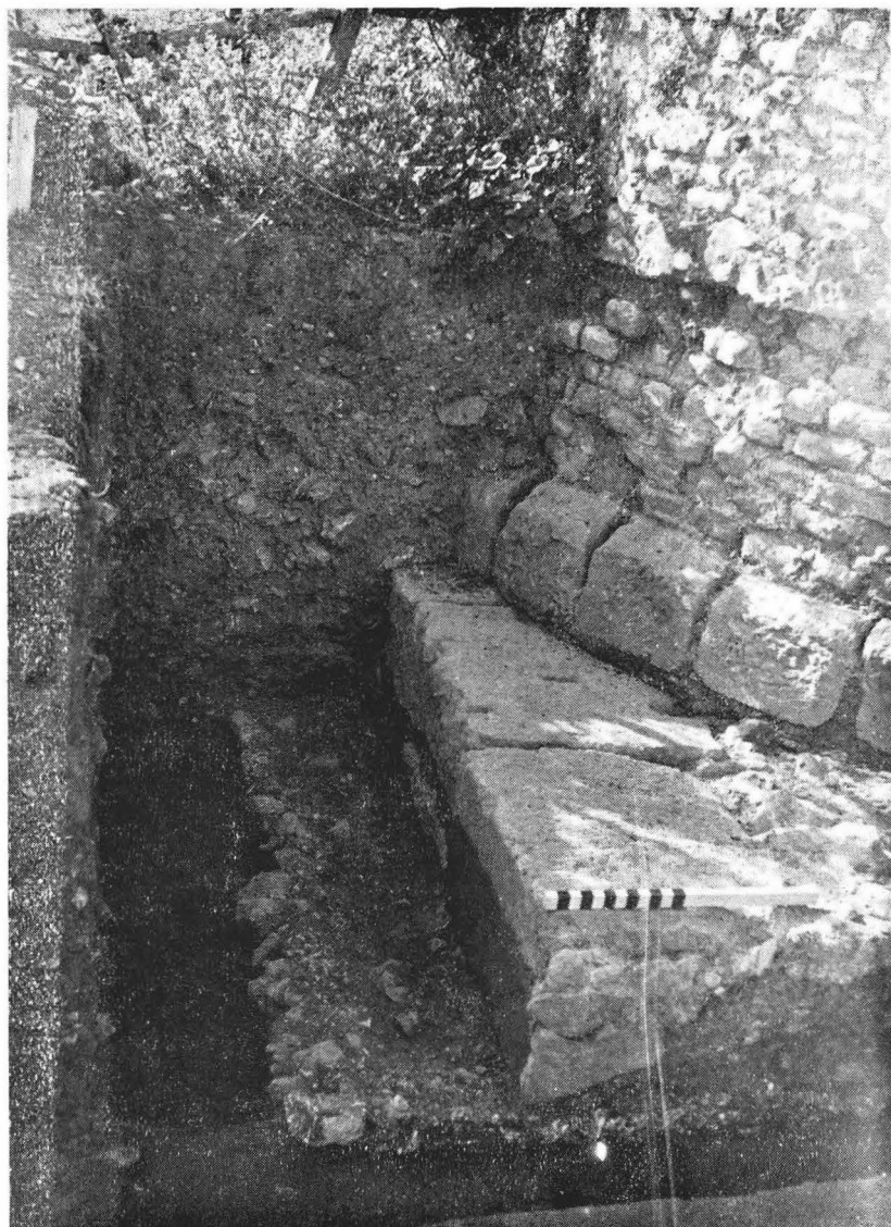
Plate II Rammed chalk foundations of bastion
