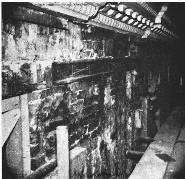
PLATE IVb. ONE OF THE PIERS BETWEEN THE MAIN WINDOWS, SHOWING THE CAST-IRON SPREADER
