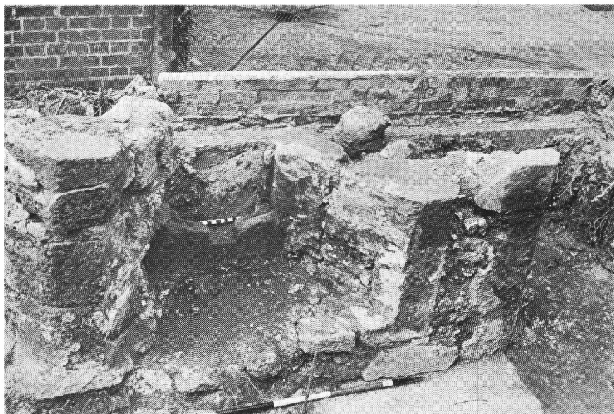
PLATE VA. West range. North section of west wall, with malthouse doorway made in an embrasure.
