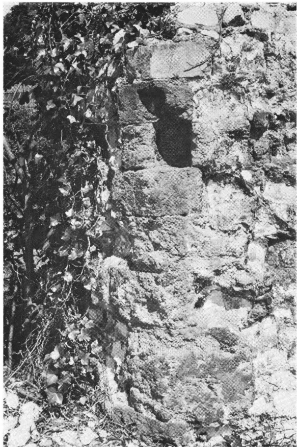
PLATE IVA. North range. Detail of doorway in the north wall. Bolt hole is 4ft above ground level.
