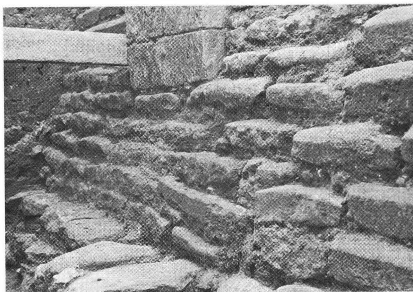
PLATE 10. Repair to west wall and foundations.
