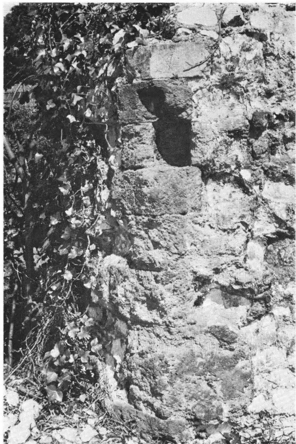
PLATE IVA. North range. Detail of doorway in the north wall. Bolt hole is 4ft above ground level.
