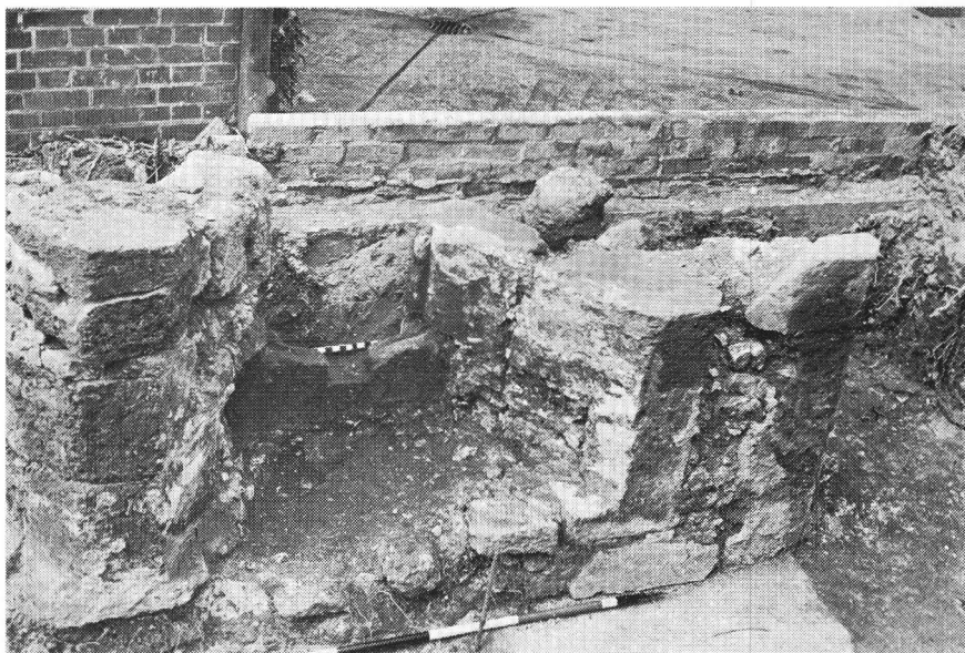
PLATE VA. West range. North section of west wall, with malthouse doorway made in an embrasure.
