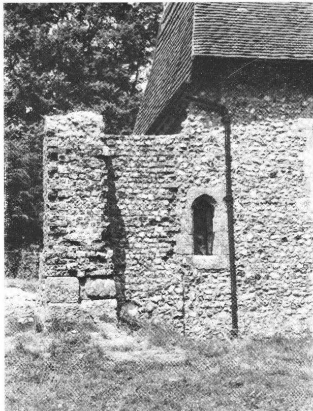
PLATE VI. Standing section of ruined walls of buildings A, B and C, from south. Immediately to the west of south-west angle of present building can be seen low side window of Building B, in green sandstone, with trefoil head and remains of iron grille. To the west of window are the chancel arch buttress and repaired section of south wall of Building C in squared
