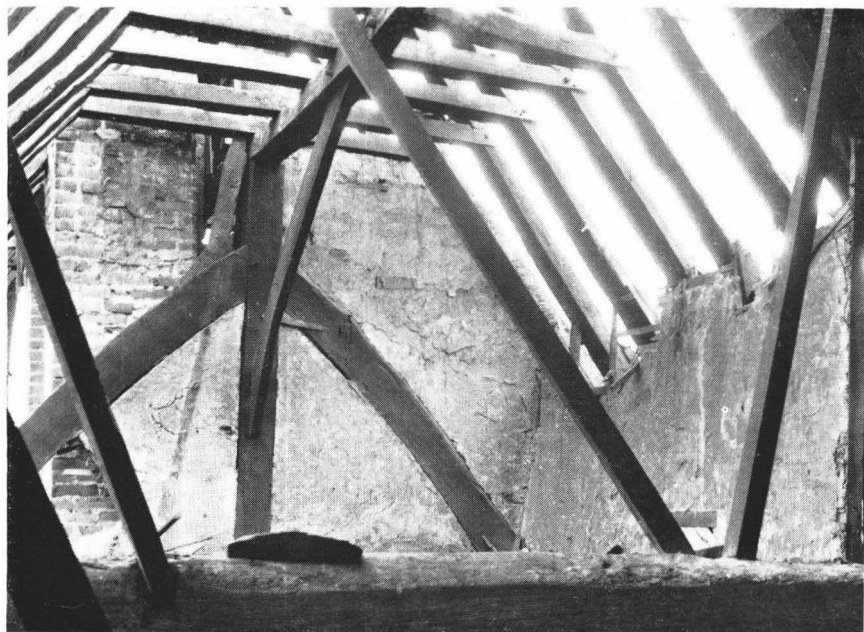
A. Roof to the open bay of the hall
