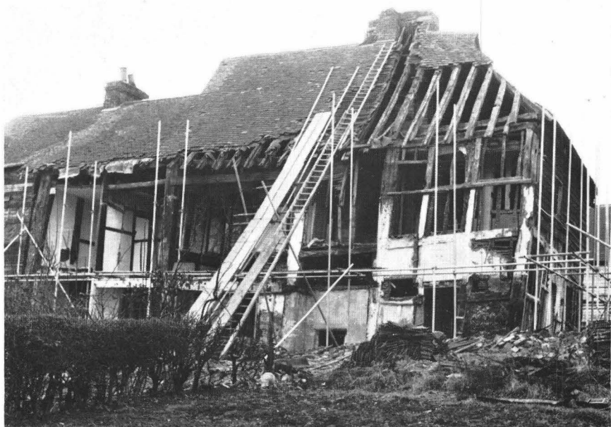
B. South elevation of building during stripping, 1968-9
