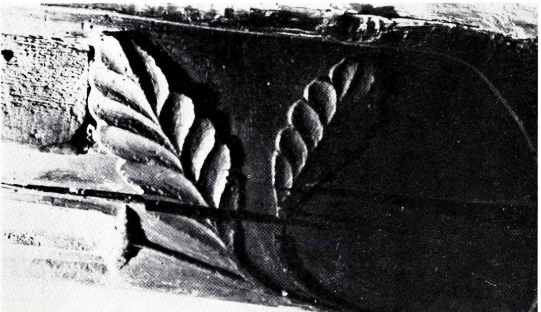
Plate II. Pope's Cottage, Hartfield. Leaf stop to dais beam, early fourteenth century
