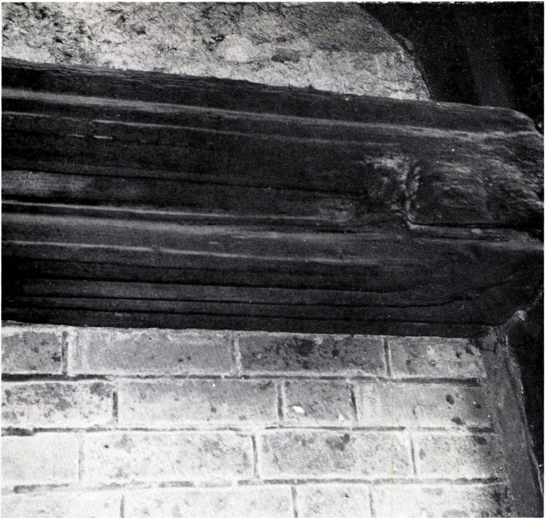
Plate I. 48 High Street, East Grinstead. Dais beam moulding, early fourteenth century. End wall of hall re-built in brick
