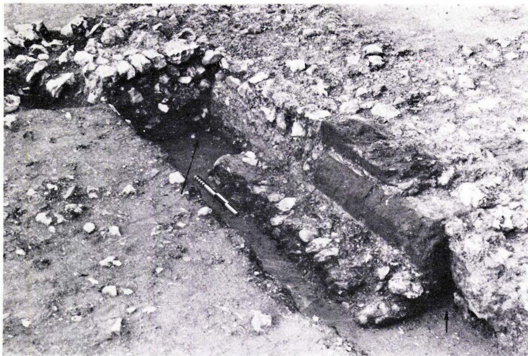
Plate III. Butt-joints between nave and chapel (short arrow), and between nave and western porch (long arrow). Scales in centimetres and decimetres
