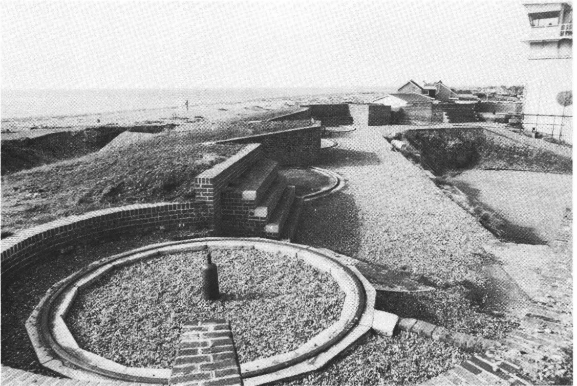
Plate III Photograph of Shoreham Fort in 1980. This shows the restored gun platform.
