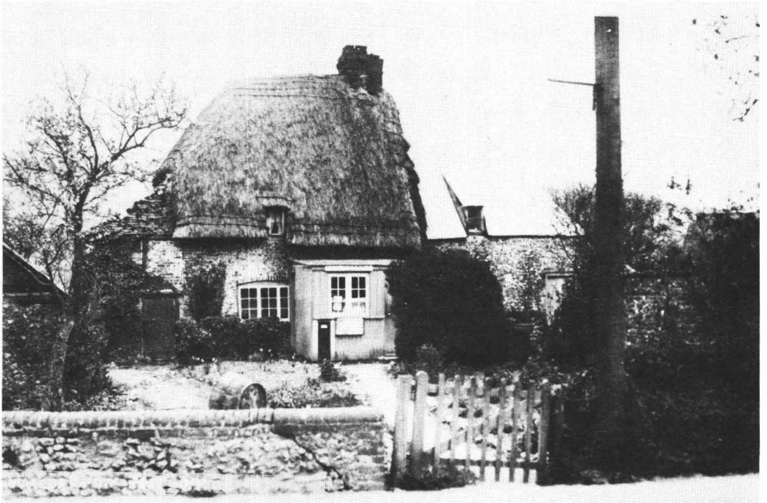
Plate II. Walderton Cottage, a view of the north side in about 1950. This shows the east outshot and the corrugated tin extension in use as a Post Office. Reproduced with the kind permission of Mr. M. Uniacke.
