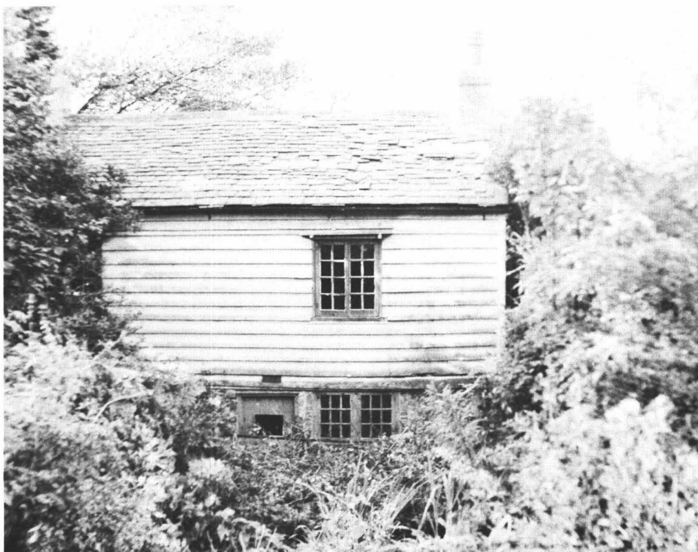
Plate II. South-east elevation of the miller's cottage, photographed in the summer of 1962, showing the basement entrance.
