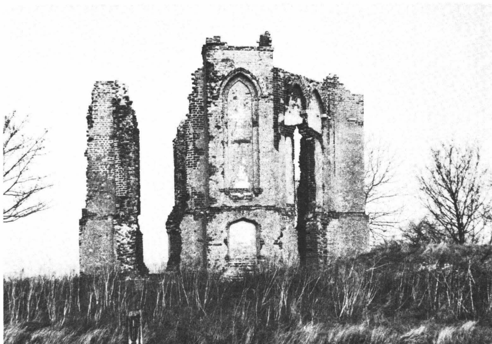
Plate 1. Vandalian Tower, Uppark, from the south-east, after consolidation in 1982.
