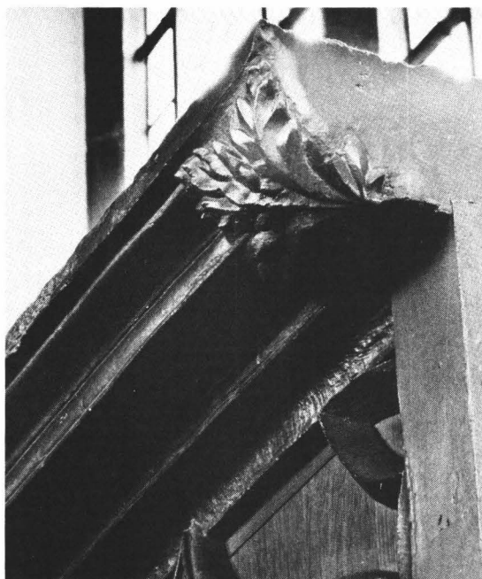
Fig. 8. St. Mary's Hospital, Chichester. Cornice termination at east end of north range of choir stalls.
