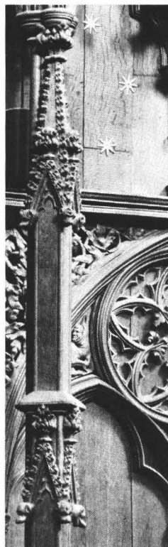
Fig. 14. Winchester Cathedral. Choir stall buttress detail.
