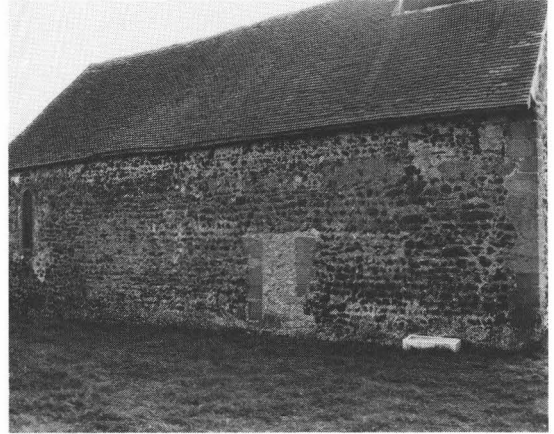
Fig. 5. Greatham Church: north wall (Photo R. Wilmshurst).
