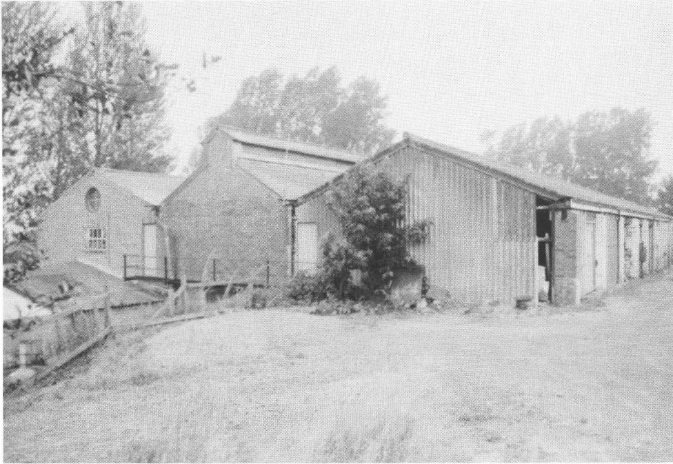
Fig. 21. Udiam Oast: Modern Kiln Roof Replaces Six Chimneys.
