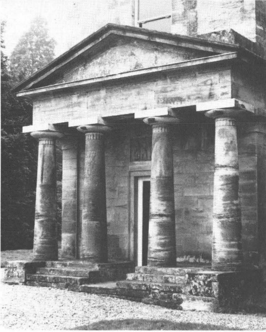
Fig. 2. Hammerwood Lodge, now called Hammerwood Park, near East Grinstead, Sussex, designed by Benjamin Henry Latrobe in 1792. This is the first, and so far as is known, the only, use in England of the 6th century BC Order of the so-called Basilica at Paestum. The capitals and abaci are of Coade stone.
