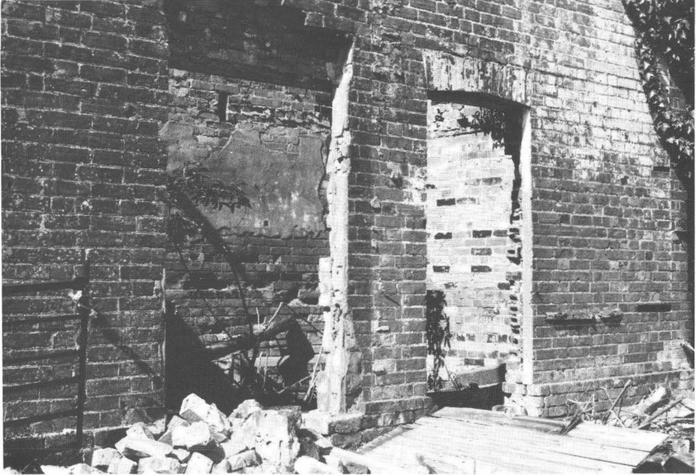
Fig. 20. Stockwood Firs Oast: Hollow Lining Bricks inside the Kiln.
