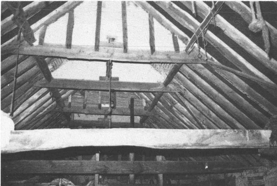
Fig. 10. Hollow Wall Oast: The Tops of the Inset Kilns in Situ.
