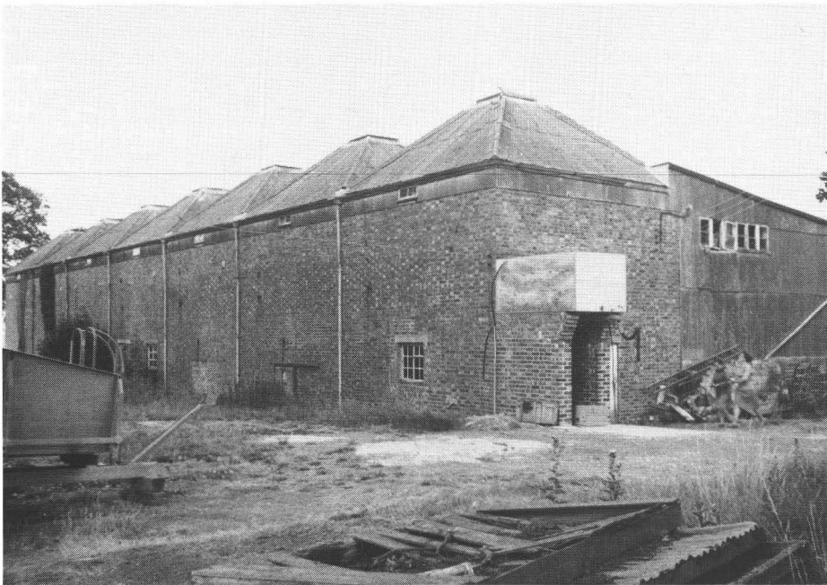
Fig. 22. Ockham oast: Seven Kiln Oast, Its Roofs Rebuilt.
