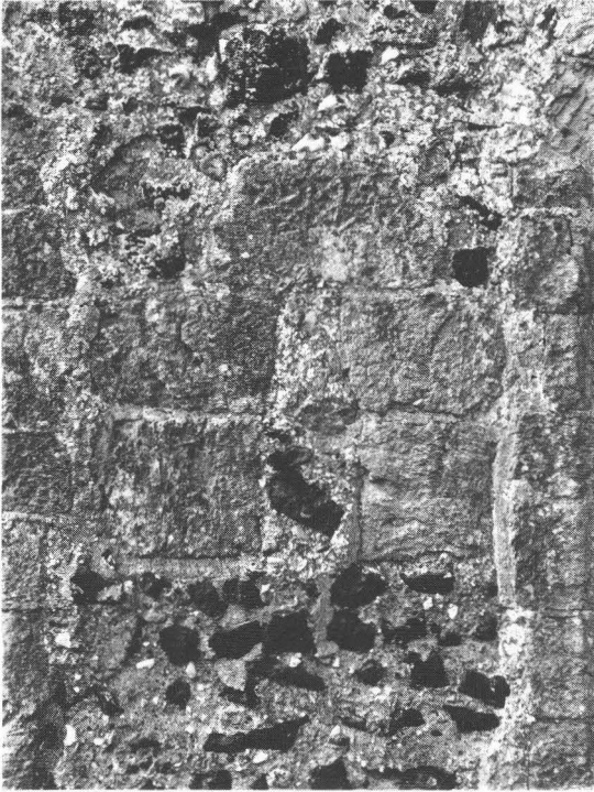
Fig. 4. Greatham Church: blocked window in east wall (Photo R. Wilmshurst).
