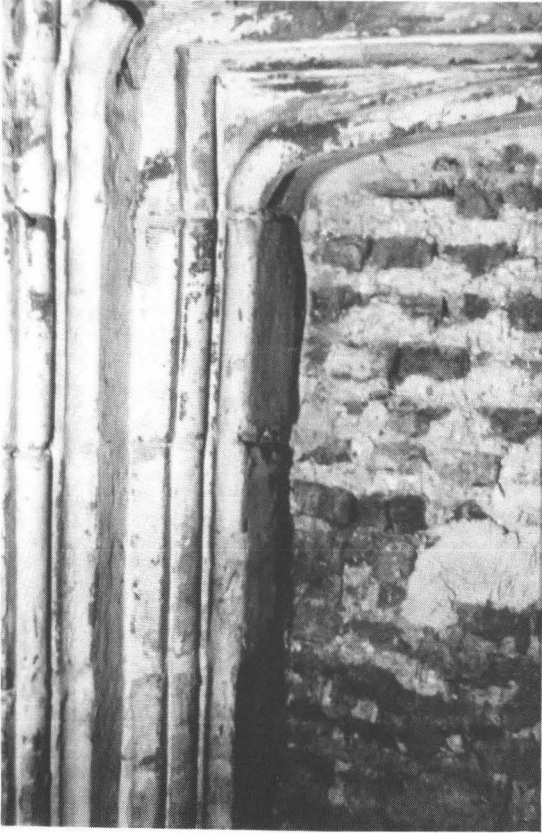
Fig. 30. Laughton Place. Internal terracotta doorway on first floor, as revealed during the 1978-81 restoration.
