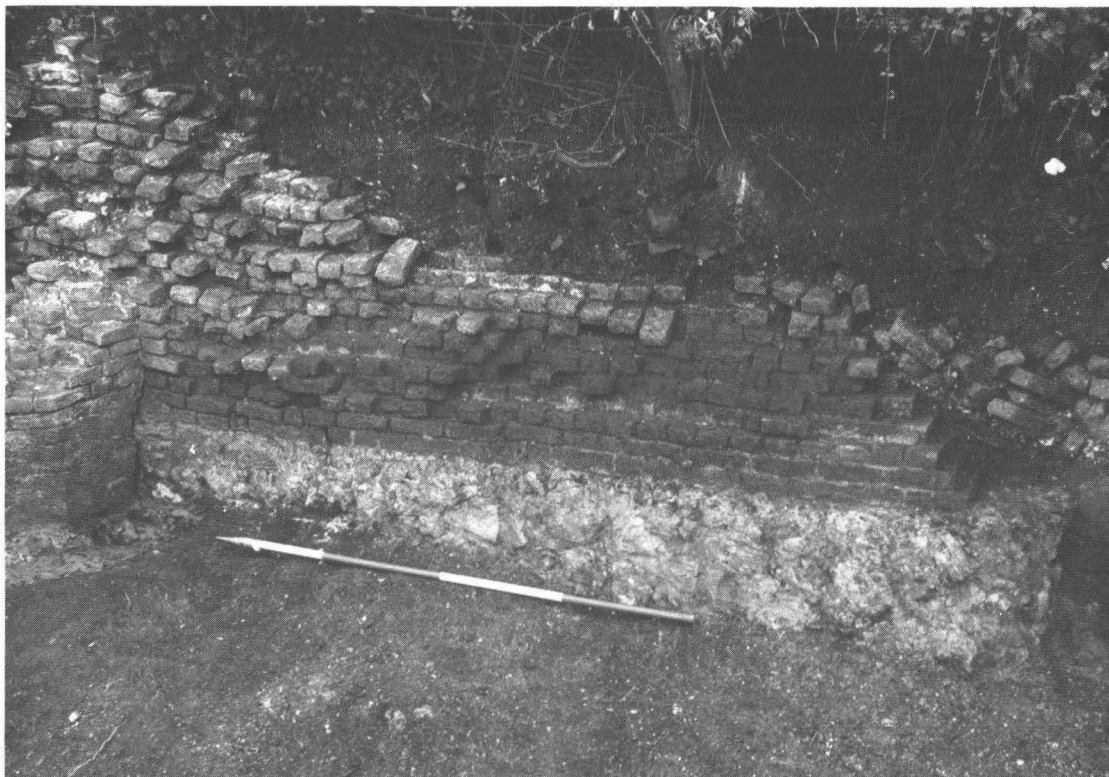
Fig. 18. Laughton Place, 1984. Tudor brick wall-projection and 'stepped' end of curtain wall. Area P. Scale: 2 m.
