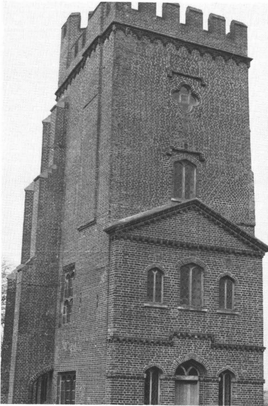
Fig. 25. Laughton Tower in its present condition showing south-east and south-west faces.
