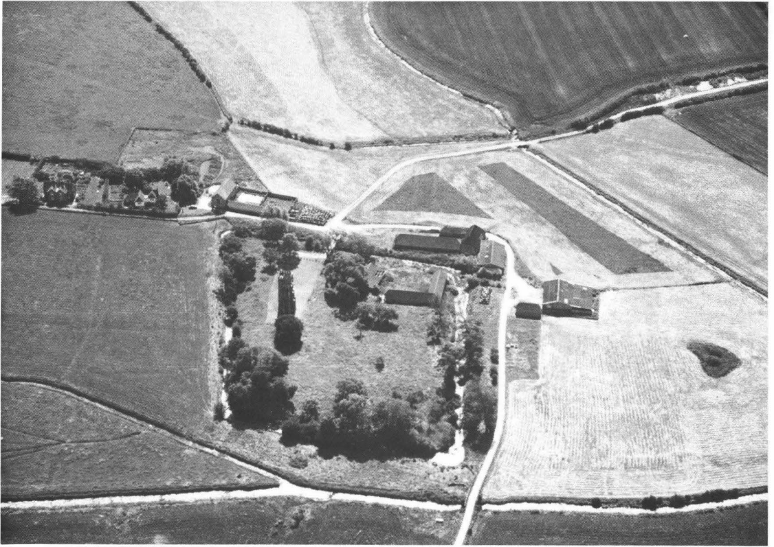
Fig. 1. Laughton Place, 1985. Aerial view from the north-west.
