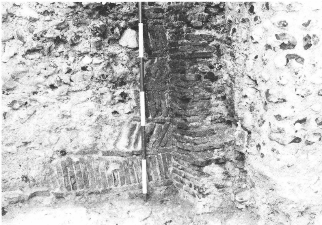
Fig. 9. Lewes Castle, 1987. Area C. Tile-backed fireplace in 13th century hall. Scale in 20 cm. intervals.
