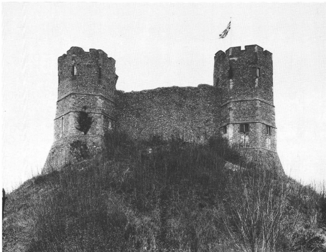
Fig. 3. Lewes Castle. Shell keep on south-western motte showing 13th century angle towers.
