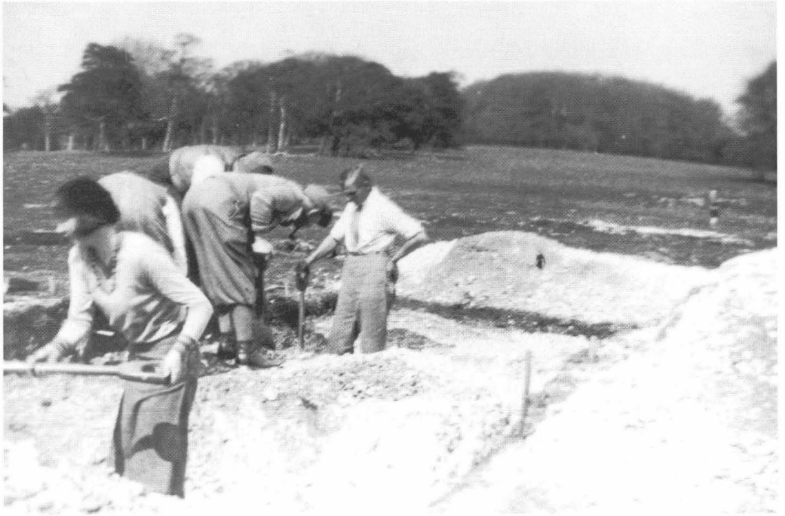
Fig. 2. Trenching in progress at Shepherd's Garden, Arundel Park.
