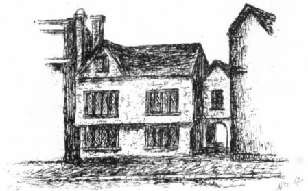
EAST FRONT OF WEST WING. No. 4
