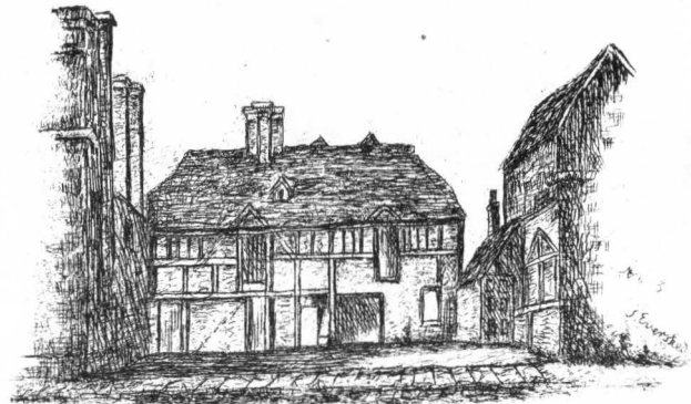
WEST FRONT OF EAST WING. No. 3
