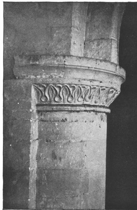
CAP. OF EAST RESPOND OF NAVE ARCADE; S. SIDE.
