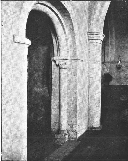
EARLY-POINTED ARCH, E. END OF S. AISLE ; AND WEST RESPOND OF DECORATED CHANCEL ARCADE.
