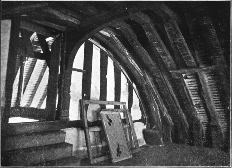
ROOF OF HALL (UPPER END).
