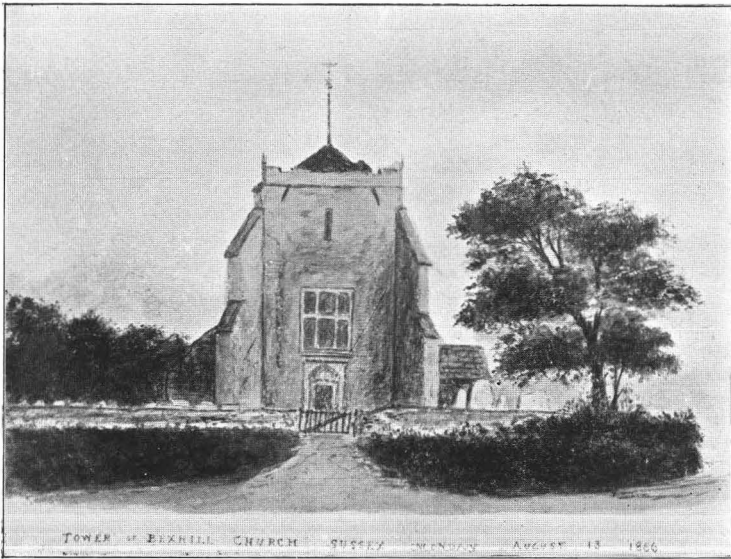
TOWER, LOOKING EAST.
