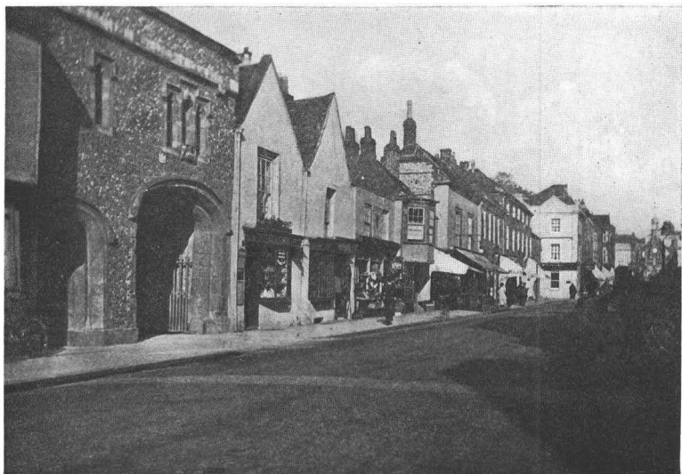
4. CANON GATE AND EAST SIDE OF VICARS' HOUSES, REFRONTED ONTO SOUTH STREET.
