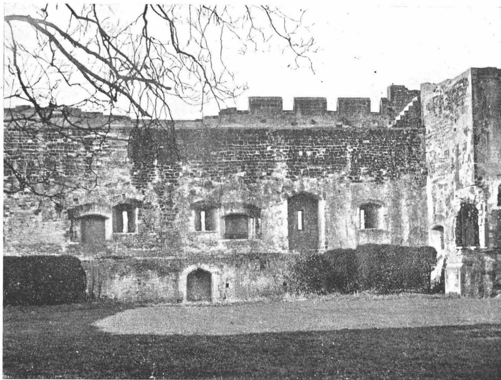
INNER SIDE OF WEST CURTAIN WALL. Showing remains of domestic buildings in upper storey.
