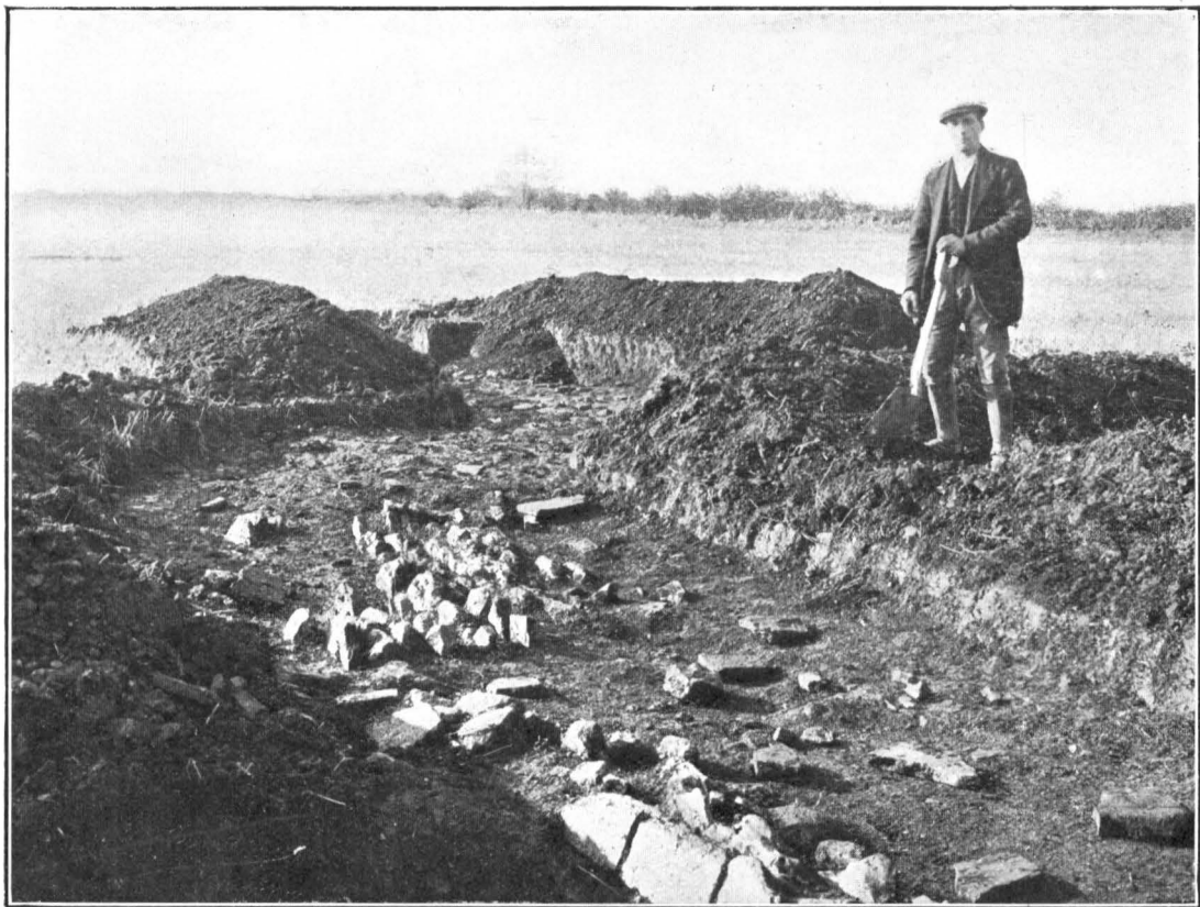
PLATE III. INTRA-VALLUM ROAD, looking South, with bend down towards fosse; showing stones and bricks set edgewise.
