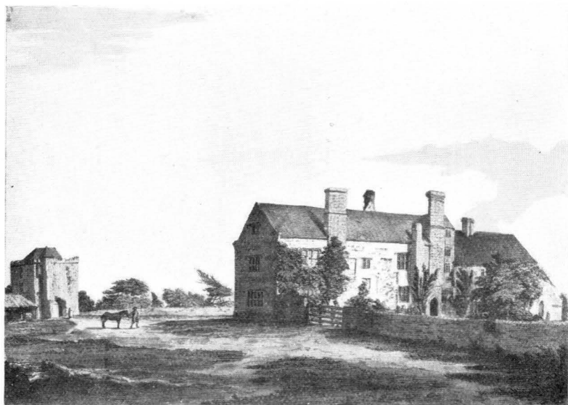
THE GATEHOUSE AND TUDOR WING, FROM THE SOUTH.
