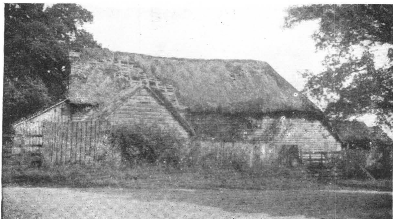
STONEHOUSE BARN, SOUTH SIDE.
