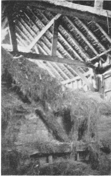
STONEHOUSE BARN, INTERIOR LOOKING NORTH WEST.
