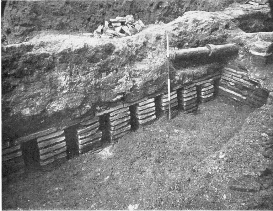
FIG. 7. ROOM III: HYPOCAUST PILLARS RECESSED INTO WEST WALL.
