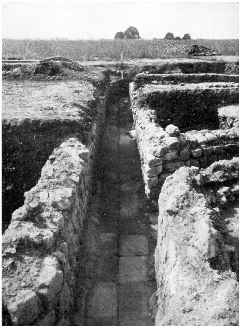
FIG. 19. MAIN DRAIN SEEN FROM THE NORTH. SUB-DRAIN ENTERING FROM COLD PLUNGE BATH ON THE RIGHT.
