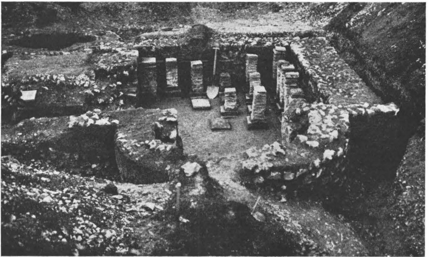
FIG. V. THE HOT ROOM (from the East).
