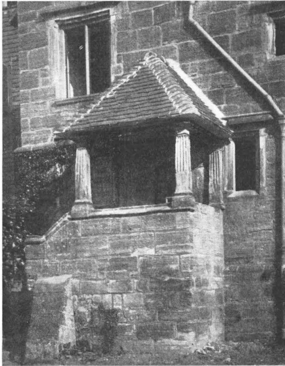
FIG. 10. PORCH HOUSE: THE PORCH.
