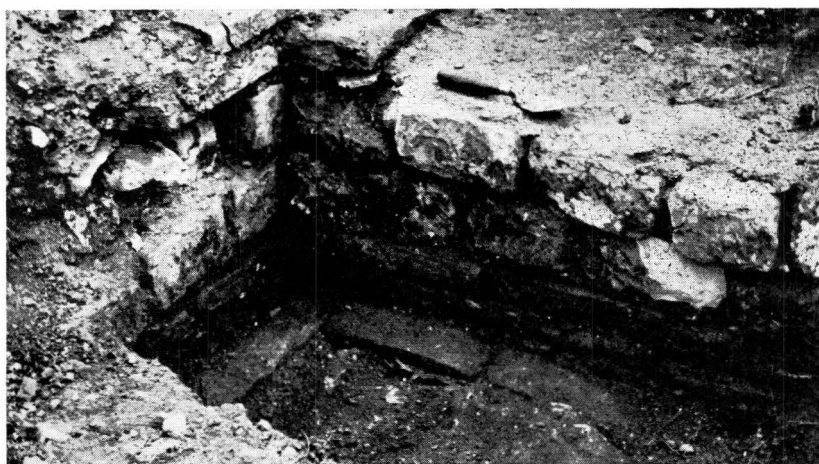
2. Inner Face of North-east Corner
