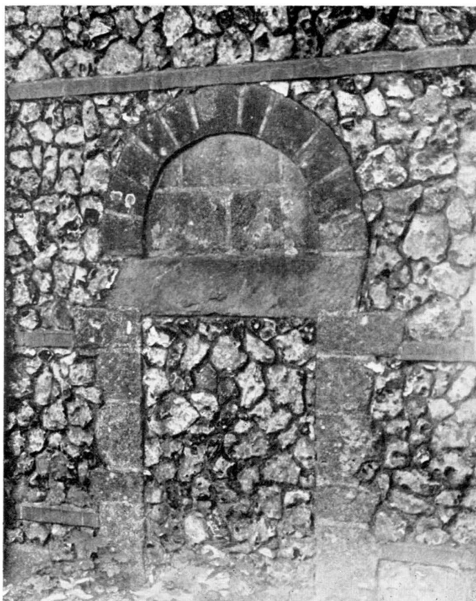
PLATE VII. PATCHAM: BLOCKED NORTH DOOR
