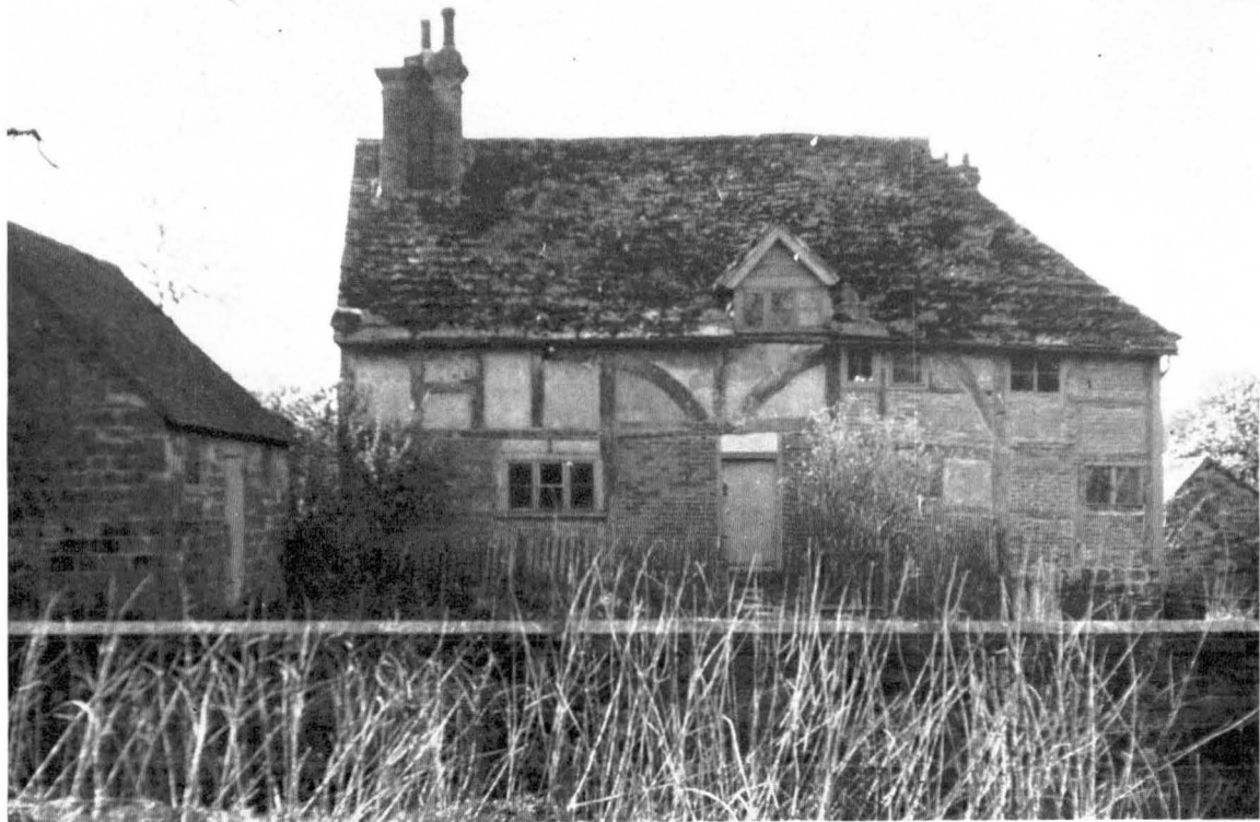
PLATE I. BELL'S FARM: NORTH SIDE; HALL AND BUTTERY BAYS
