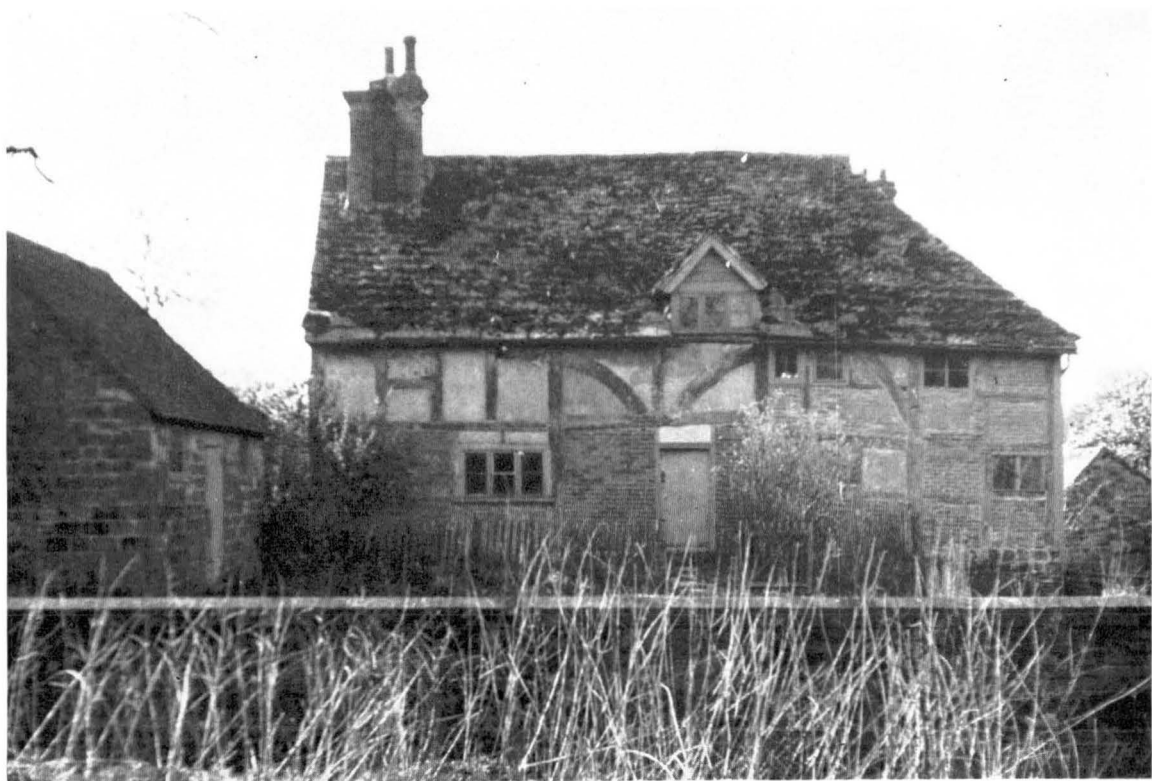
PLATE I. BELL'S FARM: NORTH SIDE; HALL AND BUTTERY BAYS
