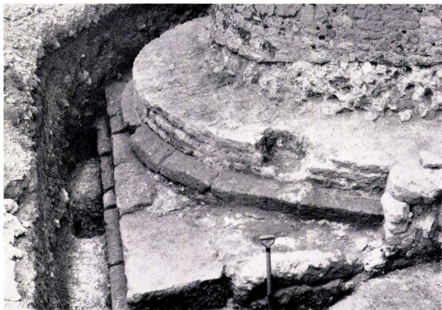
PLATE III. FOUNDATIONS OF MARKET AVENUE BASTION (see Fig. 7)
