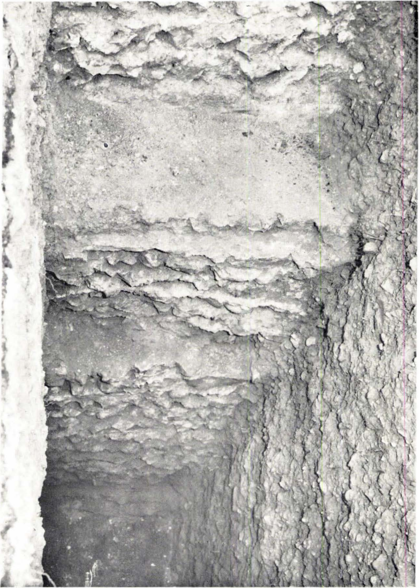
PLATE I. INNER FACE; ROMAN WALL: North Walls (see Fig. 1, G)
