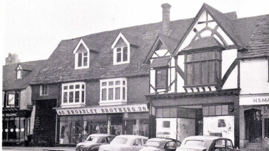
PLATE VIII. NOS. 36, 38, AND 40 HIGH STREET, EAST GRINSTEAD. The fourteenth-century Hall is on the left
