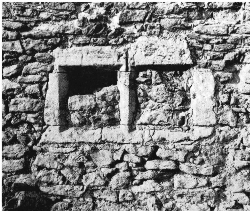
PLATE III. DOUBLE WINDOW OPENING in north wall of Becket's Barn, August, 1956
