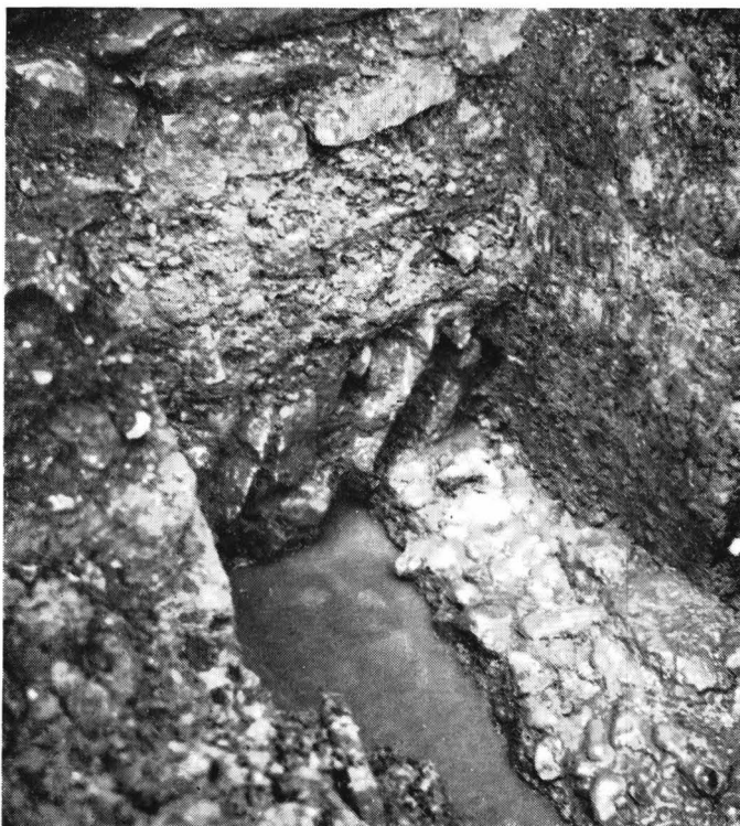
PLATE V. CUTTING ON NORTH SIDE OF BARN showing cobble floor, possibly late Saxon in date, December, 1956
