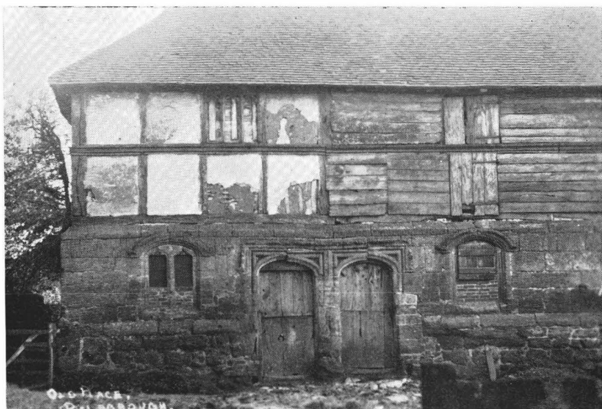
PLATE IB. OLD PLACE. View of part of building from north before demolition.
