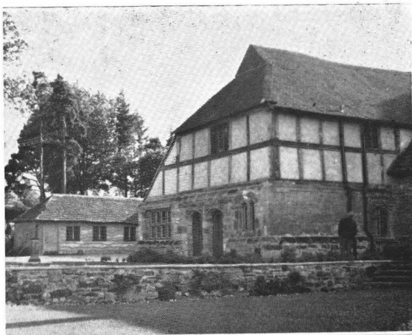
PLATE VA. OLD PLACE View from north-east after demolition and alteration
