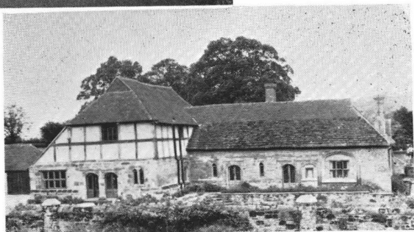
PLATE VB. OLD PLACE View from east after demolition and alteration
