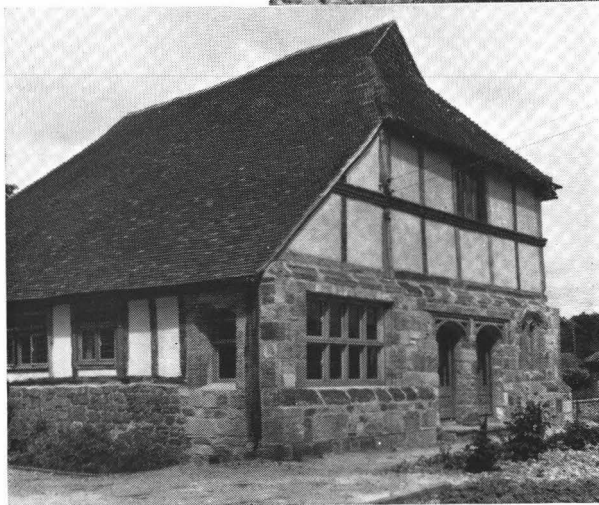
PLATE VC. OLD PLACE View from south-east after demolition and alteration
