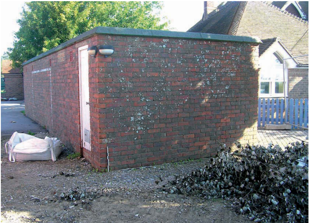
Fig. 2. The Shelter. Looking north. 9 am.
